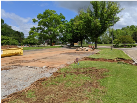
Parking lot expansion/accessible parking project at church.
