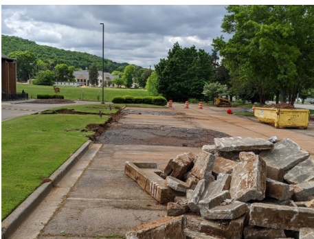
Looking south, old curb removed to create more parking spaces.
