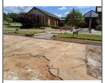
Parking lot sidewalk removed and forms in place for a parking lot level sidewalk to be poured. There will be two handicapped spaces on either side of the new sidewalk and the visitor spaces relocated on the front row.
